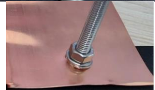
No Screw thread at hole
